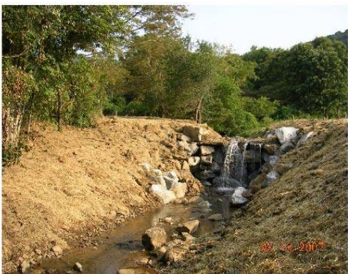
A view of the new barrier from the downstream side.
